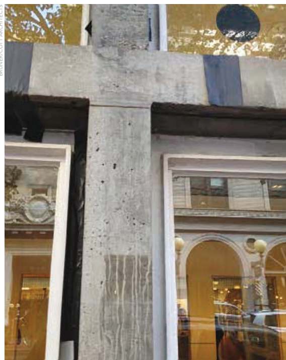
Pictured: concrete cleaning samples
